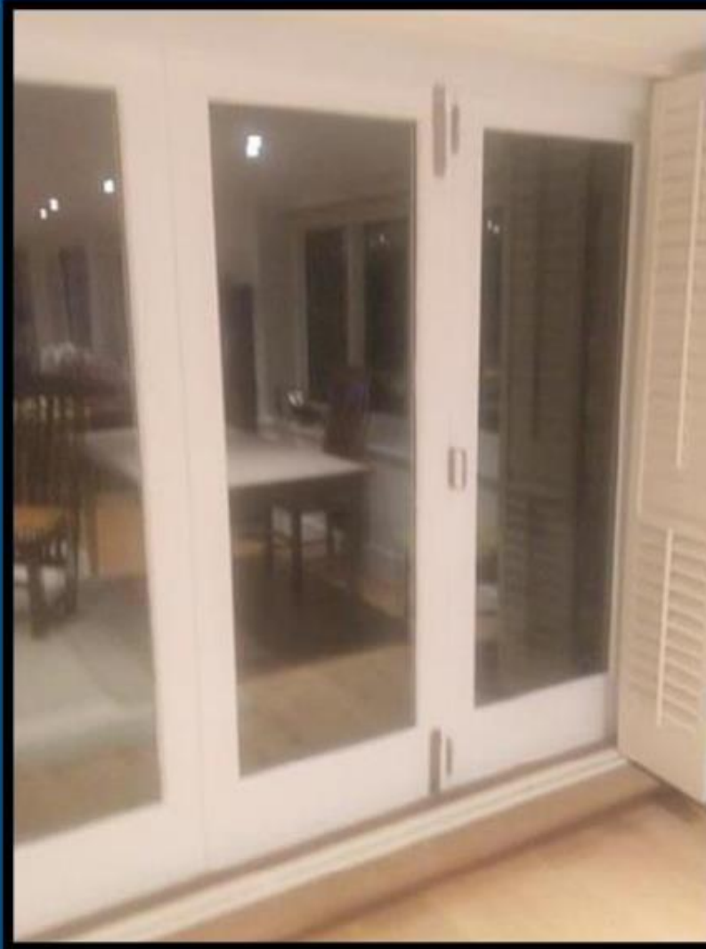
Example 4 – French doors, uneven break between door frame and door.
