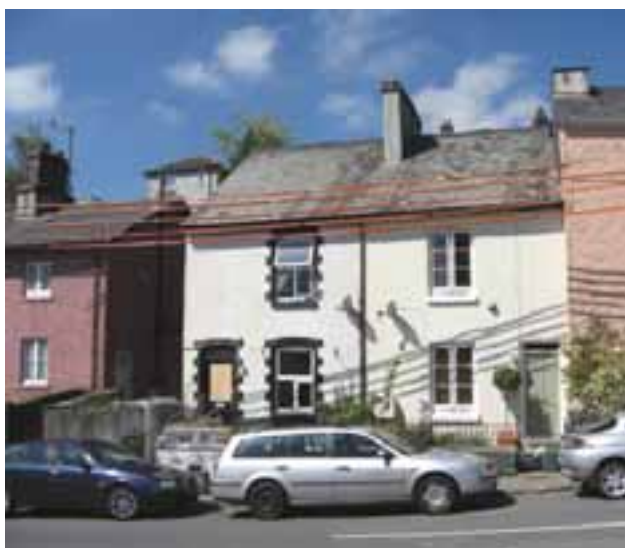
An Article 4 Direction would help to protect these unlisted houses in Bannawell Street from unsympathetic alterations
