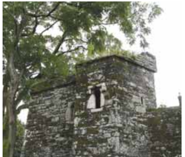
Repairs are urgently needed to Betsy Grimbal's Tower
