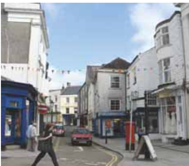
Repairs are needed to these buildings in Market Street
