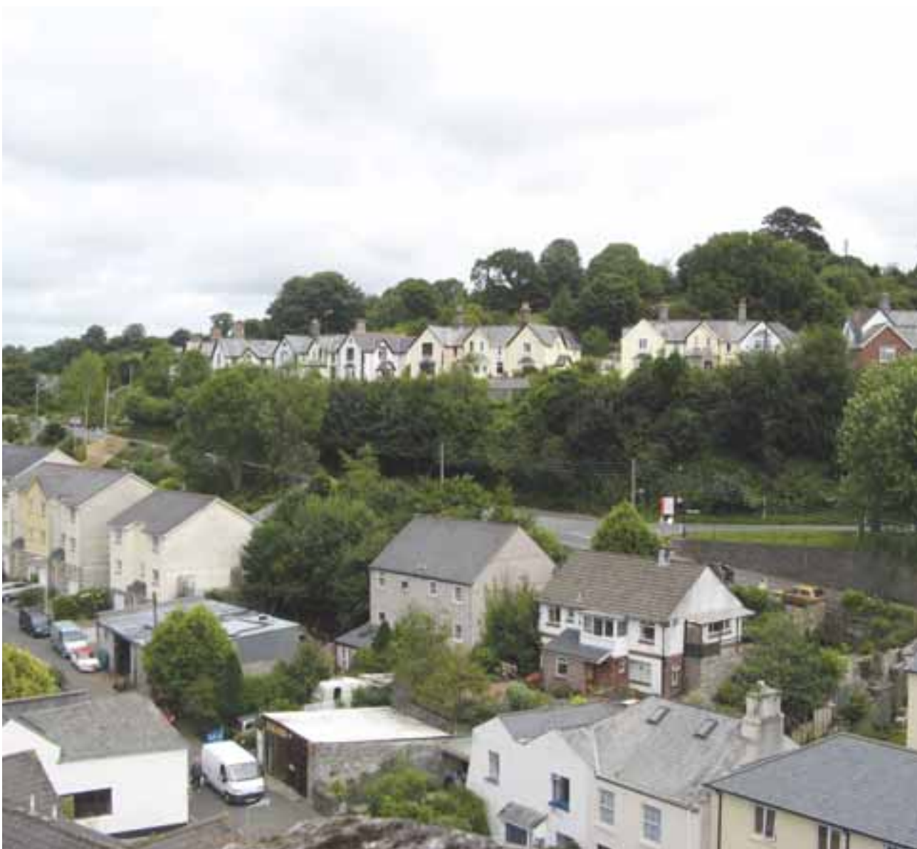
View from the railway viaduct towards Trelawny Road
