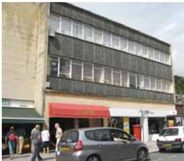
The redevelopment or enhancement of this site in Duke Street would be welcome
