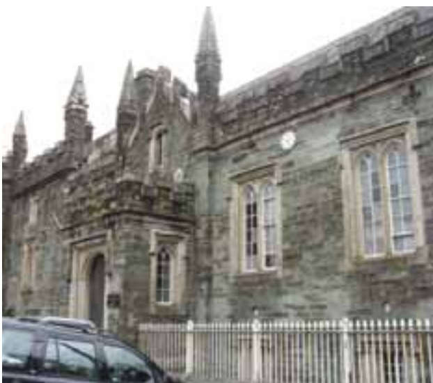
The Guildhall is already showing signs of deterioration
