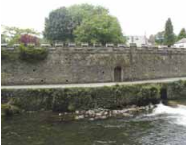
South Precinct wall
