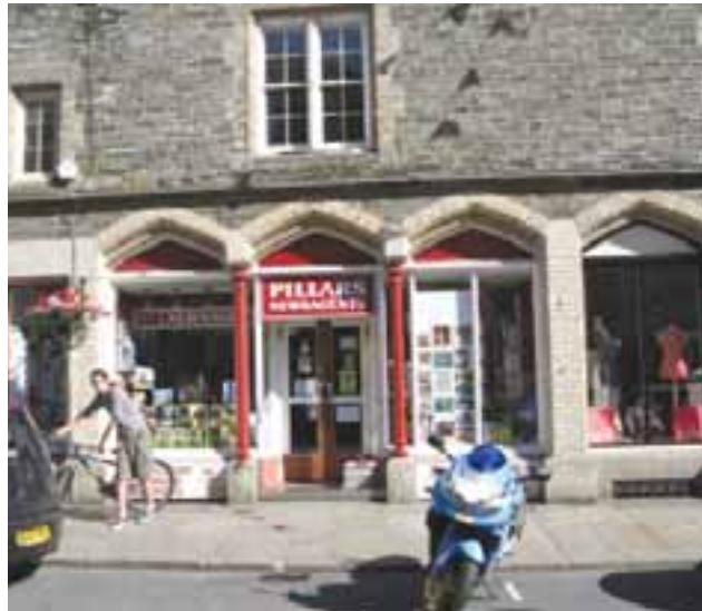
Simple original shopfront facing Duke Street
