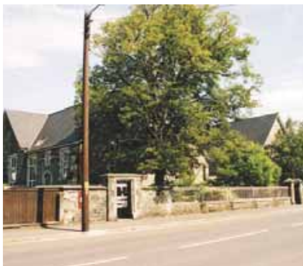
Former County Primary School, Plymouth Road
