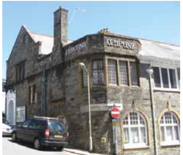
Former Tavistock Printing Company building, Pym Street
