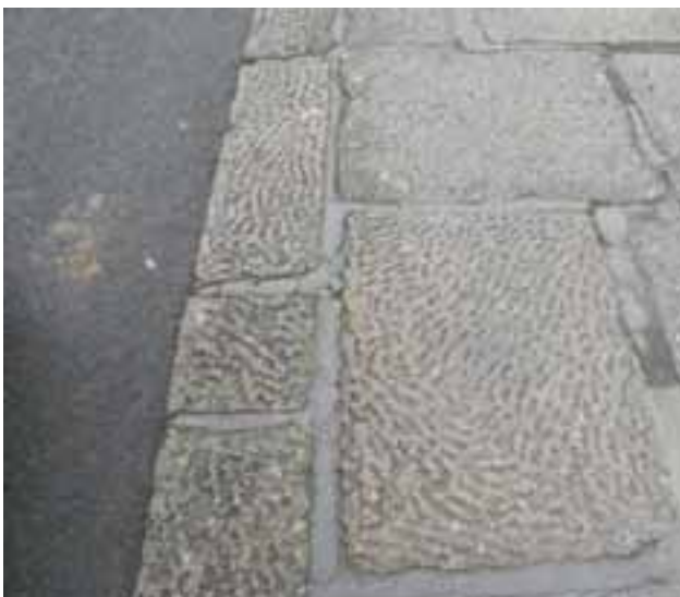
Detail of tooling on granite paving (Russell Street)
