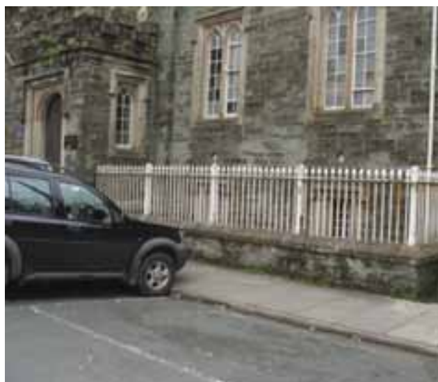
Cast iron railings outside the Guildhall
