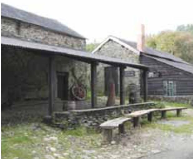
Morwellham Quay buildings
