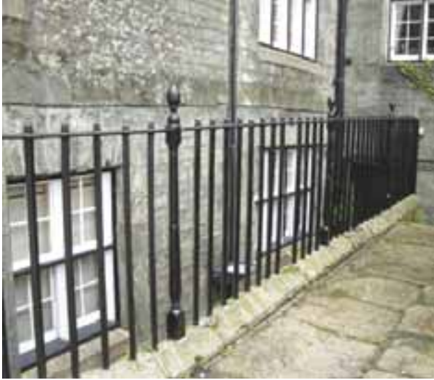
The Bedford Hotel showing ground level below street level
