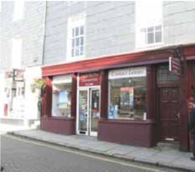
An historic shopfront in Market Street
