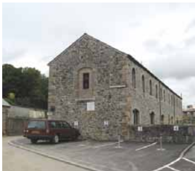
Former Upper Foundry, Parkwood Road
