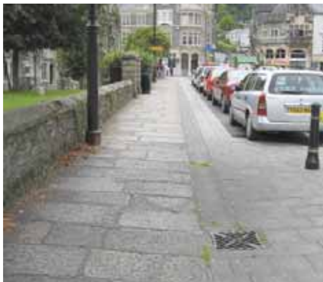
Historic and modern granite paving next to St Eustachius Churchyard
