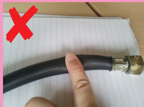
The pipe is leaking gas - the piping can be compressed and has widened. It should be firm and the same width throughout.
