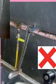
Restraining wire attached to the pipework
